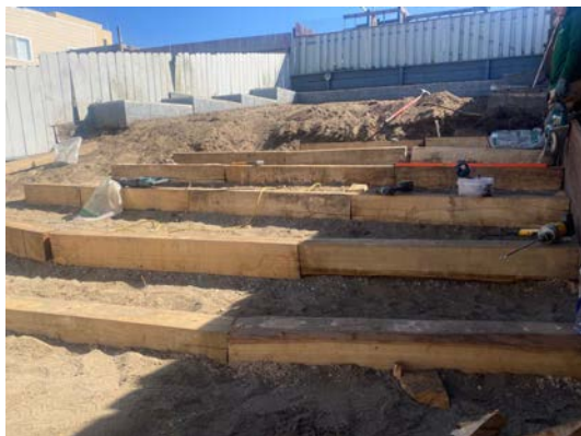
Installing tiered stairs for Deng, Qixia Daycare
